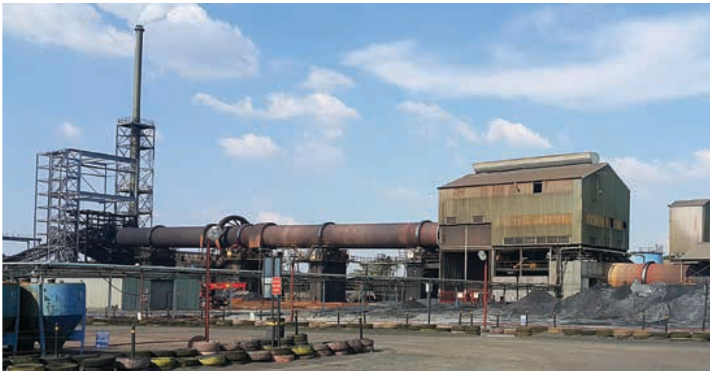
The rotary kiln, a key part of the Vametco plant.
